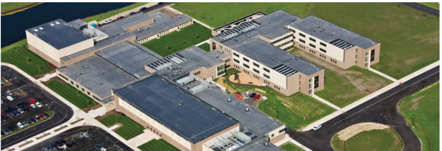
Woodstock Community Unit School District 200, New High School, Additions & Renovations
